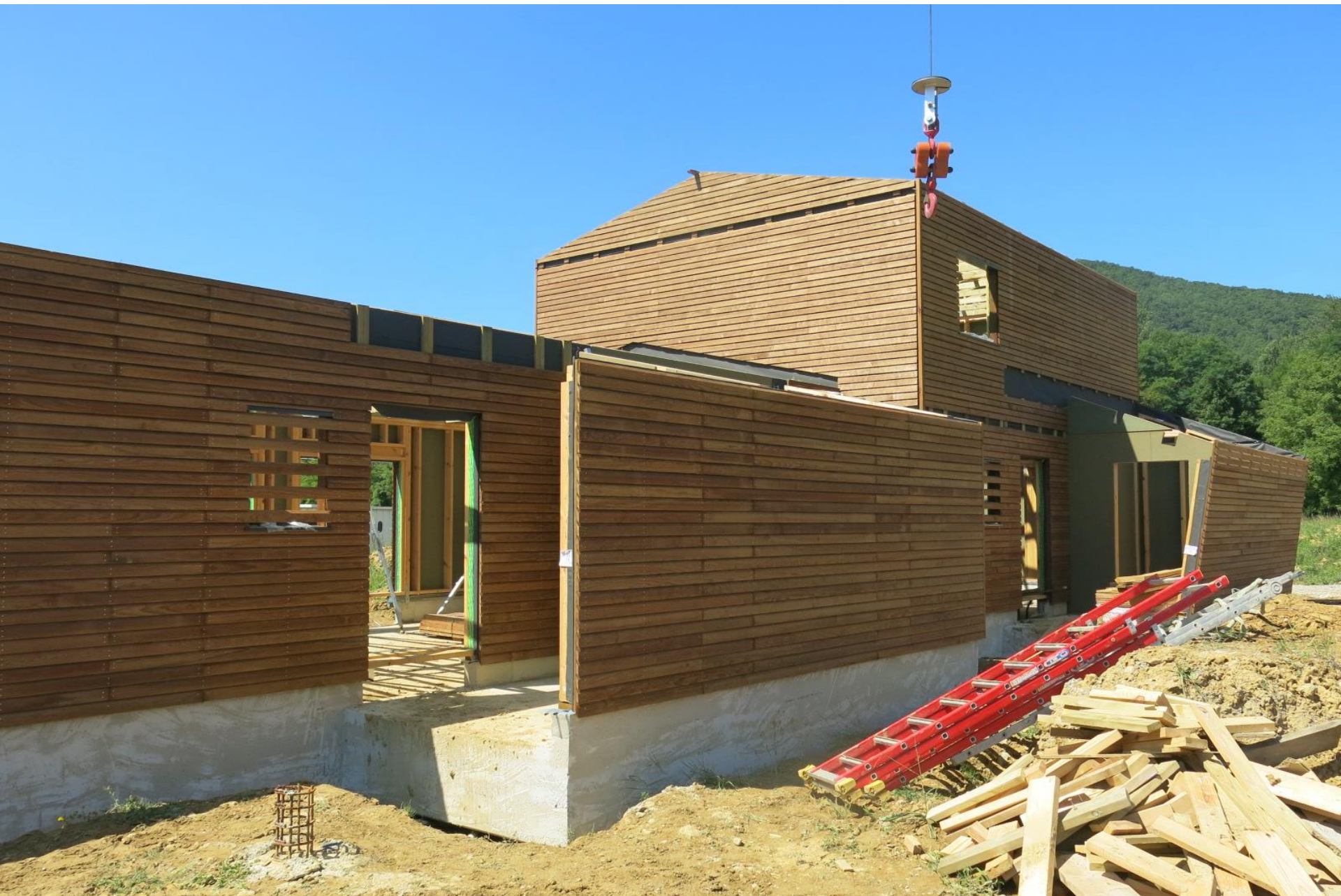
Bardage bois – menuiseries bois – plancher bois
